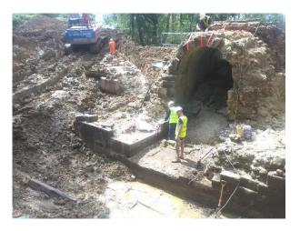
Once the wall had been dismantled with all the facing stone being carefully numbered and recorded, the barrel archway carrying the spillway (the old water control for the working furnace) was revealed. The archway was underpinned and longitudinal anchors installed. Anchors stitching together the wing walls were also installed.
