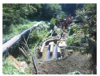
At the northern works the walls to the wheels pits were re-instated and all walls were capped. The damaged section of the tail race was also rebuilt using only stone and bricks recovered from the stream bed downstream.
