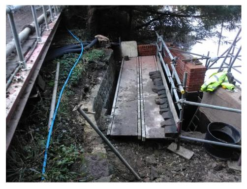
Again, at the North, the parapet wall to the 'sump' is having the top course of stones re-set. The new weir wall can be seen on the pond side (left).
