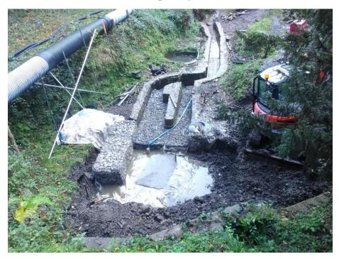
At the Northern works area the tail race is complete and gabians are being installed.
