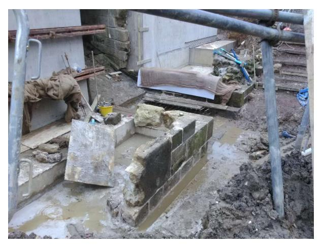
The old stonework begins to rise at the southern end. It will be a slow process as the line mortar being used takes a long time to 'go off' in cold temperatures. The original mortar was analysed and this is the closest we can achieve today.
