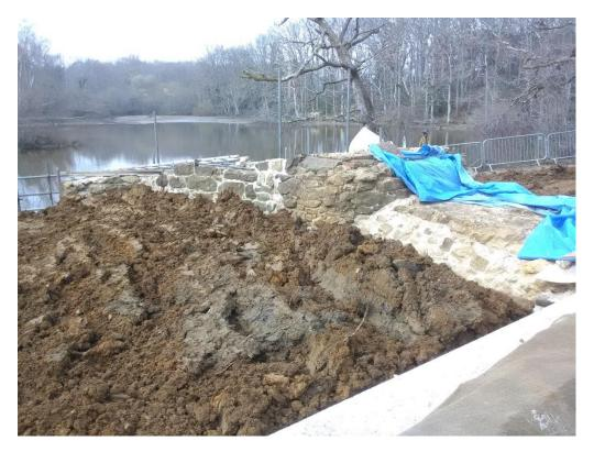
Back filling behind the new concrete wall is well under way. Thankfully the weather has remained pretty dry but earlier trying to consolidate wet clay was a difficulty. Despite the compaction a certain amount of settlement is expected.
