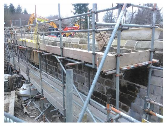
The old stonework on the southern wall has all been replaced. Some new stones were required to be cut as part of the ach to the barrel archway. The scaffolding should be coming down during the first week of April.
